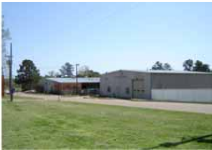
Dan Watson Building and Harris Transportation Building
