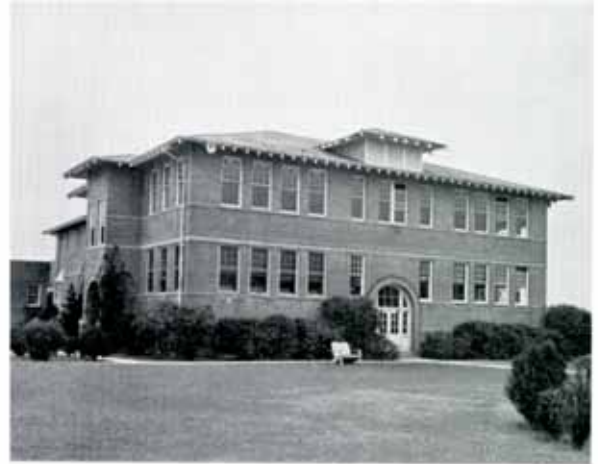
OLD ADMINISTRATION BUILDING
